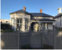
22 Auburn Grove, Armadale
