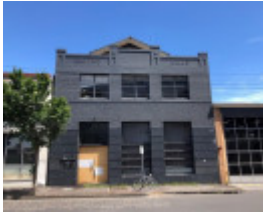
174-176 Albert Street, Windsor
