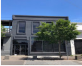
180-182 Albert Street, Windsor
