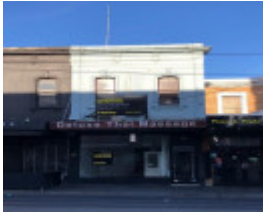
13 Chapel Street, Windsor
