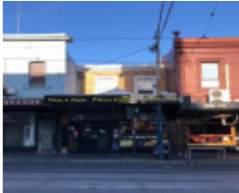
15 Chapel Street, Windsor
