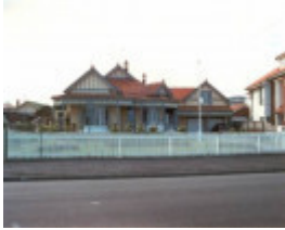
House at 89 Esplanade WILLIAMSTOWN, Hobsons Bay Heritage Study 2006
