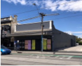
30-32 Chapel Street, Windsor
