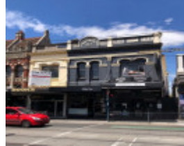
34-38 Chapel Street, Windsor
