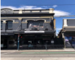
34 Chapel Street, Windsor
