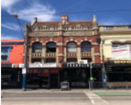
40 Chapel Street, Windsor
