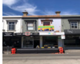
46-48 Chapel Street, Windsor
