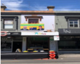
46 Chapel Street, Windsor
