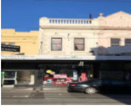
47 Chapel Street, Windsor
