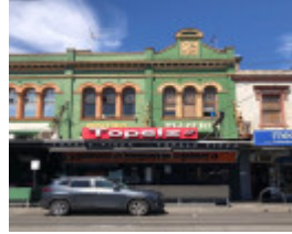
54-54A Chapel Street, Windsor
