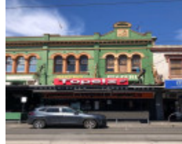
54-54A Chapel Street, Windsor
