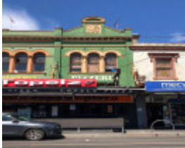
54 Chapel Street, Windsor
