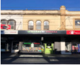
57 Chapel Street, Windsor
