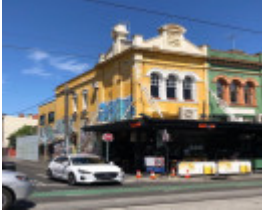
58 Chapel Street, Windsor
