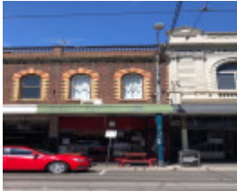
62 Chapel Street, Windsor
