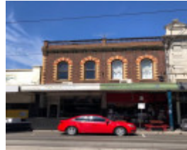
62-64 Chapel Street, Windsor
