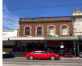
62-64 Chapel Street, Windsor
