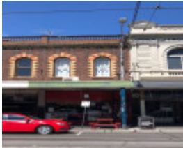
62 Chapel Street, Windsor
