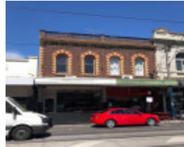
62-64 Chapel Street, Windsor
