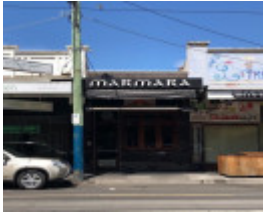
68 Chapel Street, Windsor
