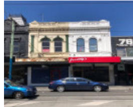
78-80 Chapel Street, Windsor
