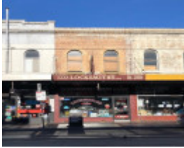
87 Chapel Street, Windsor
