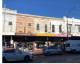
87 Chapel Street, Windsor
