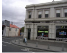
Melbourne Savings Bank (former), Hobsons Bay Heritage Study 2006
