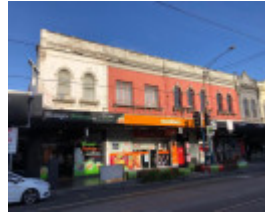
101-109 Chapel Street, Windsor
