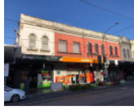
101-109 Chapel Street, Windsor
