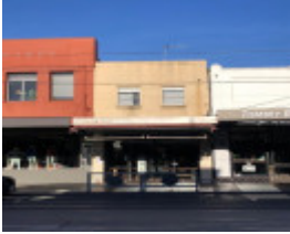
119 Chapel Street, Windsor
