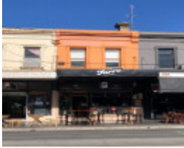
126 Chapel Street, Windsor
