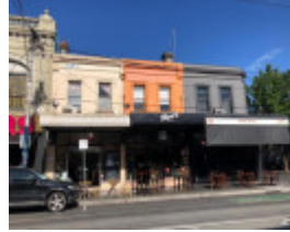
124-128 Chapel Street, Windsor
