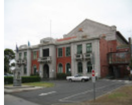
City of Williamstown Municipal Offices and Town Hall (former) and Drinking Fountain, Hobsons Bay Heritage Study 2006
