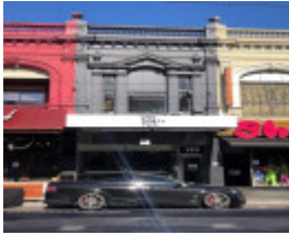
132 Chapel Street, Windsor
