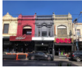
130-134 Chapel Street, Windsor
