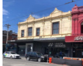
136 Chapel Street, Windsor
