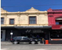
136 Chapel Street, Windsor
