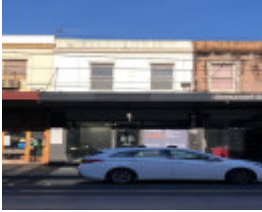
137 Chapel Street, Windsor
