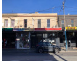
145 Chapel Street, Windsor
