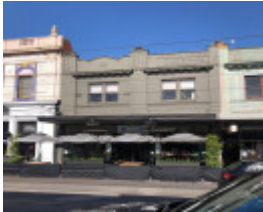
148A Chapel Street, Windsor
