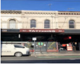
155 Chapel Street, Windsor
