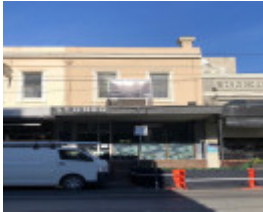
161 Chapel Street, Windsor
