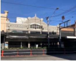
163-165 Chapel Street, Windsor
