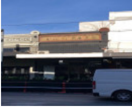
167 Chapel Street, Windsor
