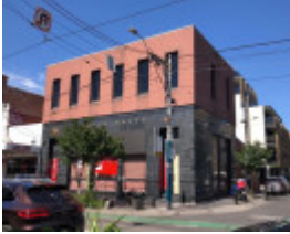
168-168A Chapel Street, Windsor
