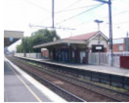
Newport Railway Station Complex and Trees, Hobsons Bay Heritage Study 2006
