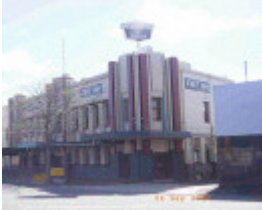
Junction Hotel, Hobsons Bay Heritage Study 2006
