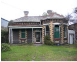
House at 184 Hall Street SPOTSWOOD, Hobsons Bay Heritage Study 2006
