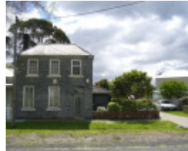
House at 6 Hanmer Street WILLIAMSTOWN, Hobsons Bay Heritage Study 2006
