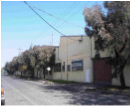
Hugh Lennon Agricultural Implements Works (former), Hobsons Bay Heritage Study 2006
