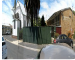
Primitive Methodist Church (former), Hobsons Bay Heritage Study 2006
