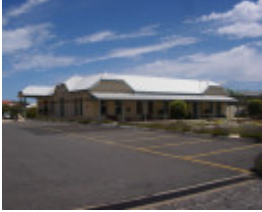
Merrett Rifle Range Pavilion (former), Hobsons Bay Heritage Study 2006
