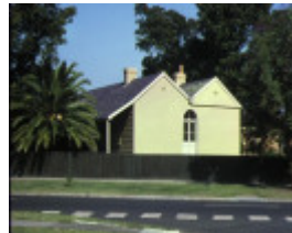
black rock house ebdan street black rock side view from street
