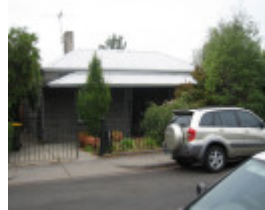
House at 9 Maclean Street WILLIAMSTOWN, Hobsons Bay Heritage Study 2006
