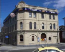
Newport Hotel (former), Hobsons Bay Heritage Study 2006
