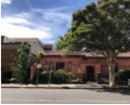
163 Peel Street, Windsor
