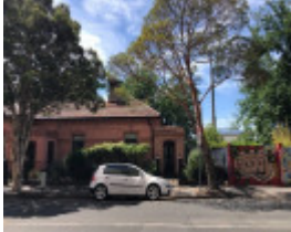
165 Peel Street, Windsor
