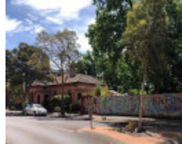
165 Peel Street, Windsor
