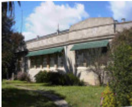
Victorian Railways Spotswood Stores Branch Complex, Hobsons Bay Heritage Study 2006
