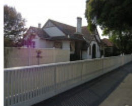
House at 278 and 280 Melbourne Road NEWPORT, Hobsons Bay Heritage Study 2006 - No 280
