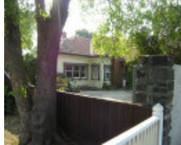
House at 278 and 280 Melbourne Road NEWPORT, Hobsons Bay Heritage Study 2006 - No 278
