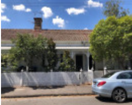
9 Beatty Avenue, Armadale
